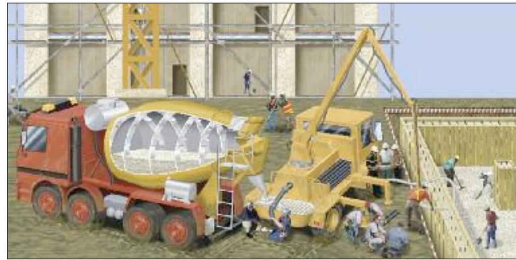
Pumping concrete from a concrete mixer into the foundations of a building (above).
