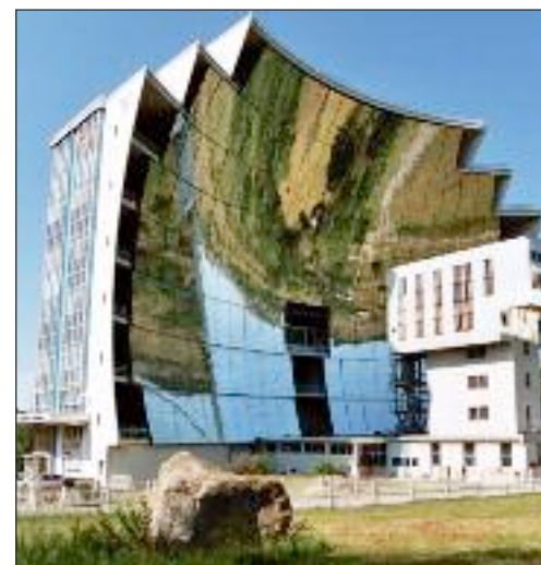
A "solar furnace", which uses mirrors to focus the sun's rays on to one spot, producing temperatures of up to 3500°C. In some furnaces, heat boils water to drive turbines and generate electricity.
